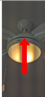
Slight wobble and noise observed at ceiling fan.
