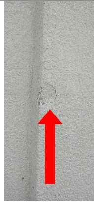
Damage to stucco by main entrance.
