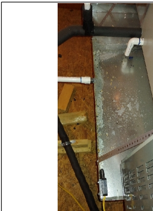
Evaporator coil has proper condensation prevention.
