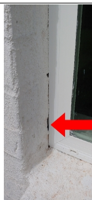
Incomplete mortar / caulking. Recommend sealing around all windows and doors.
