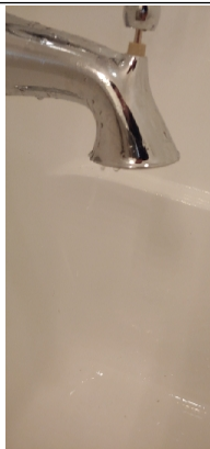
Tub faucet should NOT leak while shower is running.
