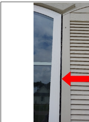
Vapor Barrier house wrap is exposed.
