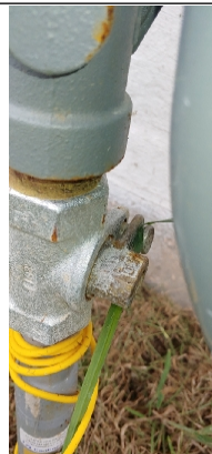
Fuel valve is locked in the off position.
