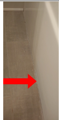
Recommend caulking to seal all openings to prevent moisture intrusion.
