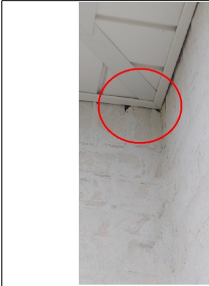
Incomplete mortar. Possible moisture and pest entry point.
