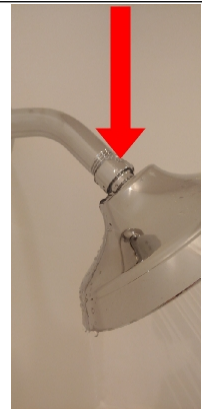
Leak observed at shower head.
