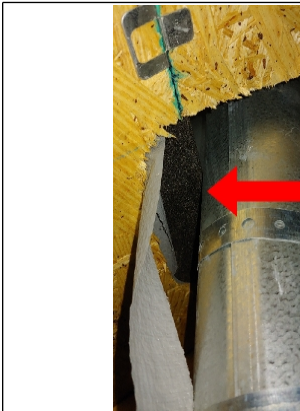
Gas B vents recommend a 1 inch clearance from combustibles.
