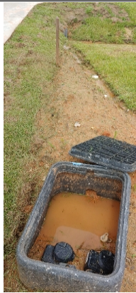
Main water shut off valve location. Information for a future homeowner.
