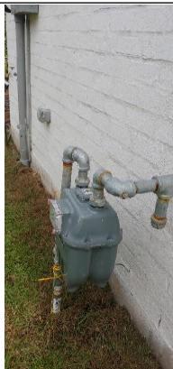
Main fuel shut off valve location. Information for a future homeowner.
